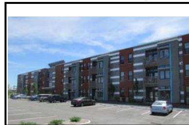
Phase I Oxford Place Senior Apartments
